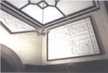
Four of the panels rescued from the East wing renovations
