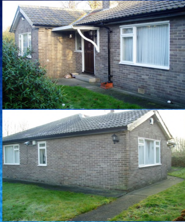
The Bungalow, Grove House
